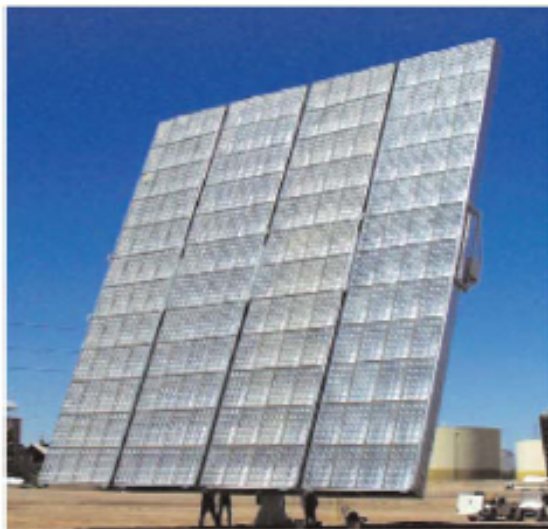
Fresnel lenses focus light on small cells: Passive cooling
